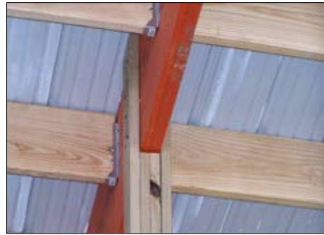
Rafter Specs, Purlin Pockets (standard)
