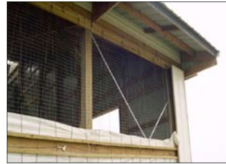
Curtain Framing 2x10 Treated Top Curtain Board (standard)
