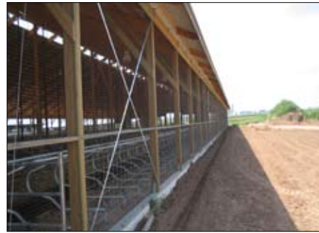
Curtain Framing, Bird Barrier, Cattle Panel Nailer, Cattle Panel Barrier (interior)
